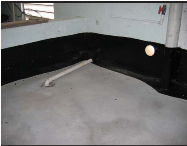
SEALING SOME MASONARY JOINTS IN A SECONDRY CONTAINMENT TANK
