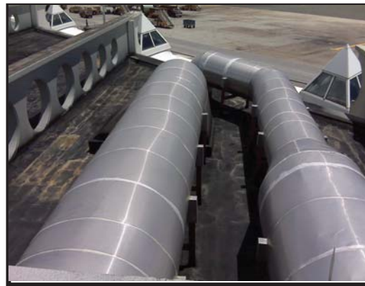
ROOF IN A FIRE HAZZARD ZONE
