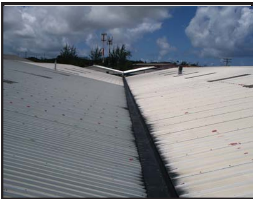
STEEL ROOF GUTTER APPLICATION
