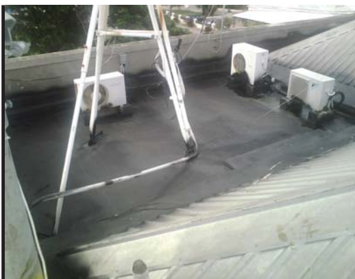
EXISTING ROOF WITH EQUIPMENT
