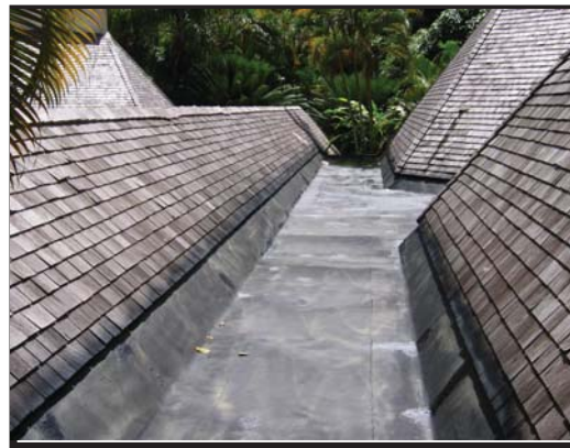
WOODEN GUTTER TO SHINGLE
